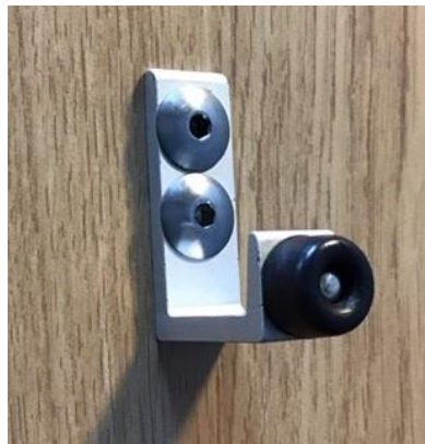
Figure 2: door buffer: ironmongery used to restrict door opening too far; fixed to either a door, floor or wall
