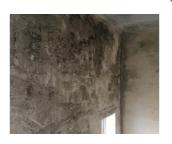
Damp refers to the presence of moisture, water and condensation being present within a property, which is often caused by condensation, penetrating damp or rising damp.
